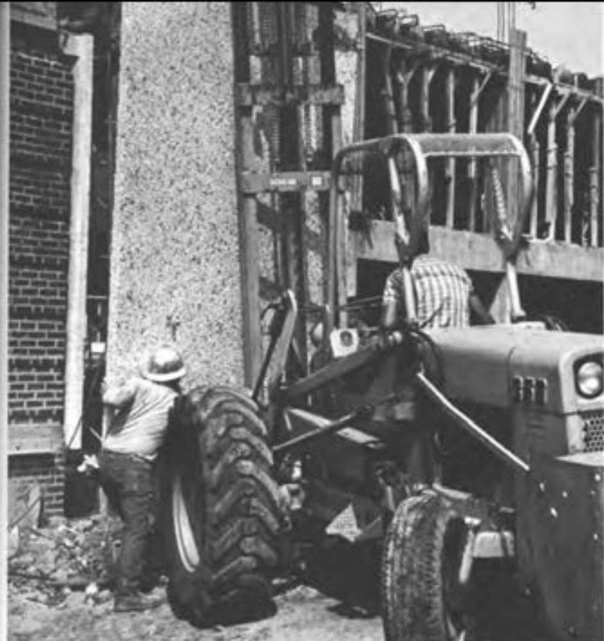
CONSTRUCTION CREW MEMBERS work on the remodeling of the science building.
